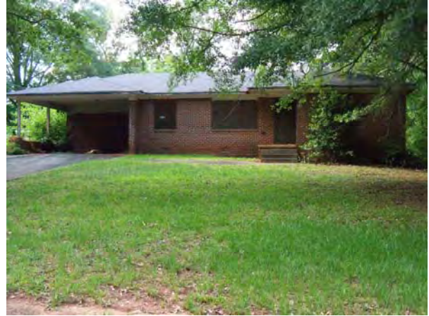
Looking North From Mellville Avenue , Subject Property
