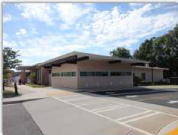
South DeKalb Senior Center to the east.
