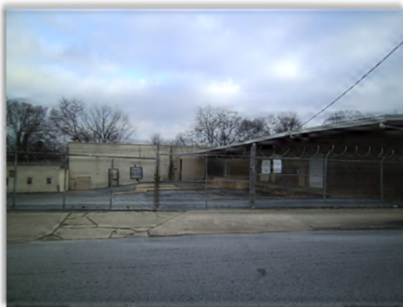
Light industrial building to the east
