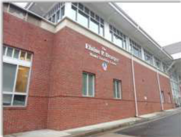
Sheltering Arms Early Education and Family Center to the south/east.
