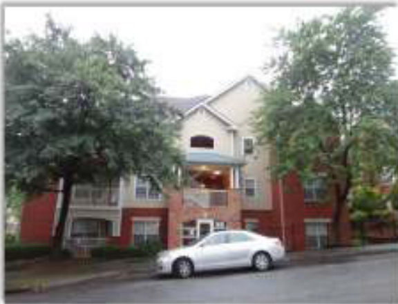
Subject building from Hunnicutt Street NW.
