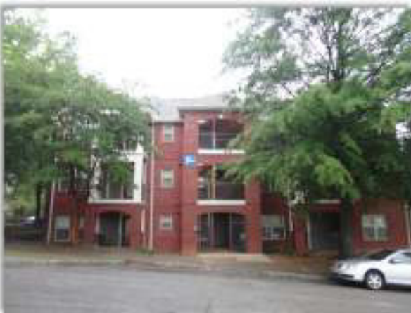
Centennial Place Phase I to the north.
