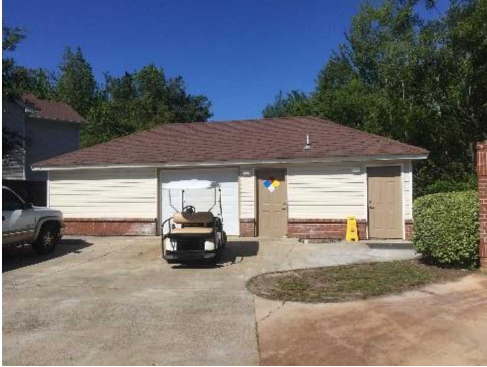
View of Maintenance Building
