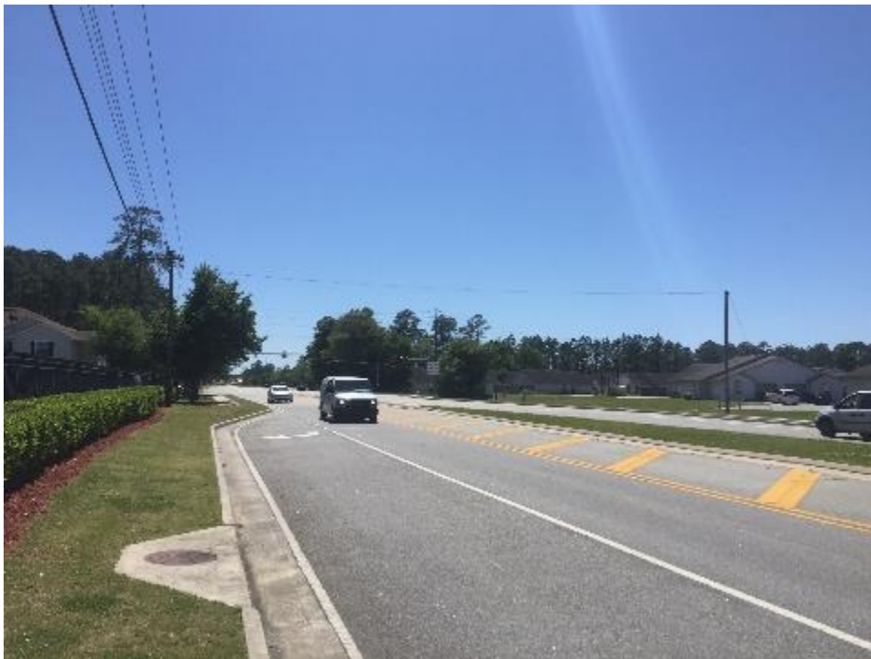
Street View of North Gross Street – To the Southwest
