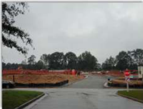
Lafayette Square Apartments, under construction to the west.
