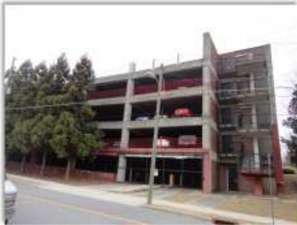
Parking deck to the west.
