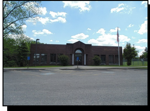
(10) Waynesboro Post Office, .3 miles west of site.
