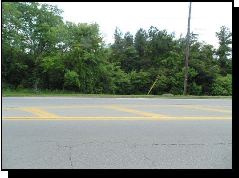
(1) Site off E 6 th Street, north to south.
