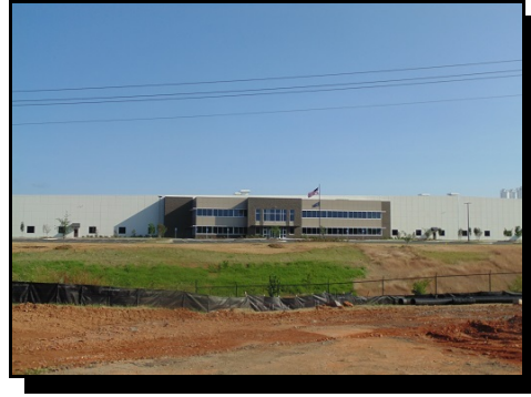
(8) Shaw Plant off GA 140, 1 mile from site.
