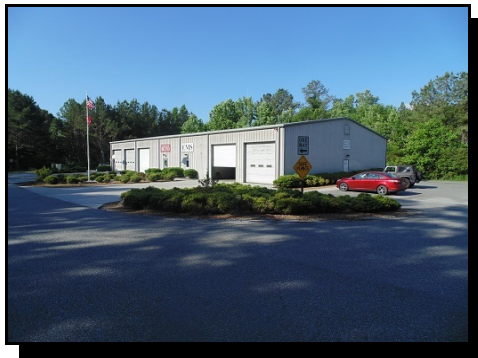
(9) EMS & Fire Station, 1 mile from site entrance.
