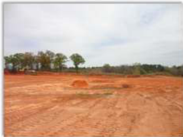
Interior of the site facing north from southern border.
