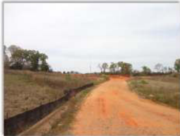
Site entrance facing west from South Houston Lake Road.
