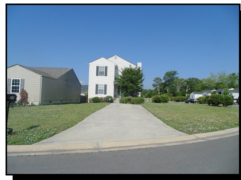
(6) Typical single-family home, south of site.
