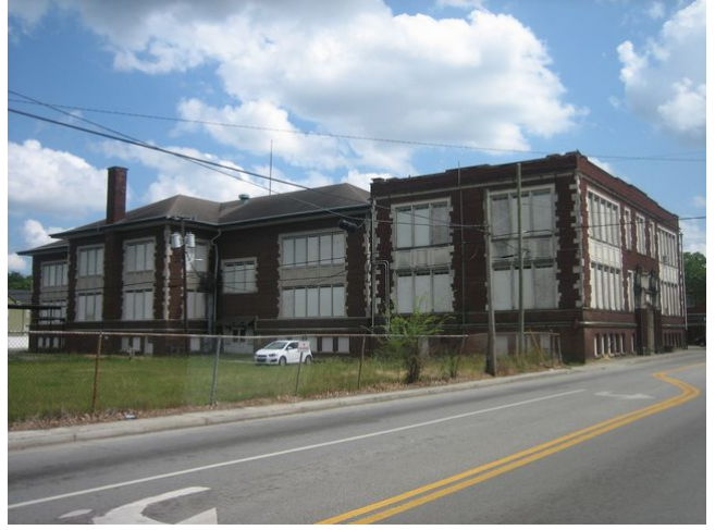
Subject (existing building)
