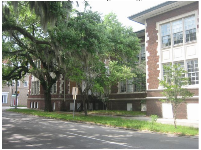
Subject (existing building)
