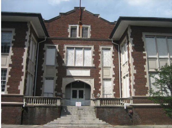
Subject (existing building)
