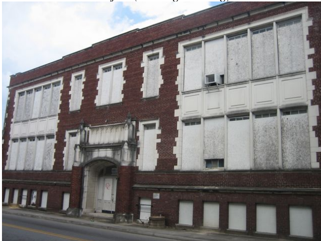
Subject (existing building)
