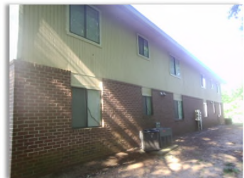
Existing residential building – rear view.
