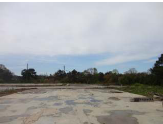
View of the site facing south from the northern border
