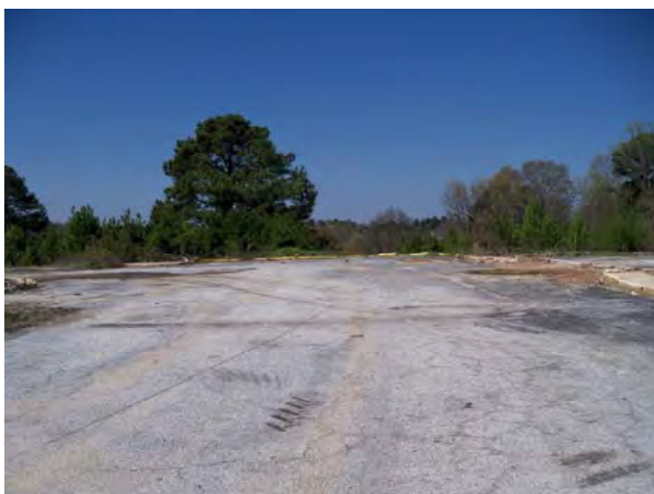
Subject Interior, Looking West
