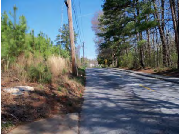
Looking North Along Hightower Road
