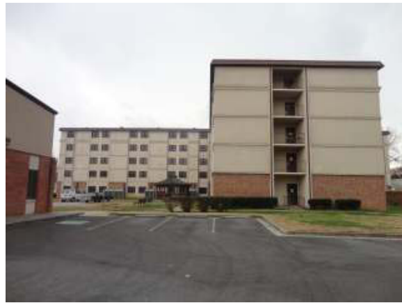
Subject building facing south
