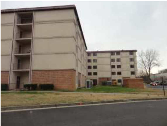
Subject building facing south
