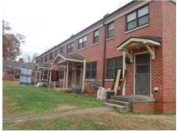
Townhouse units at Canal Court (AMP 1)
