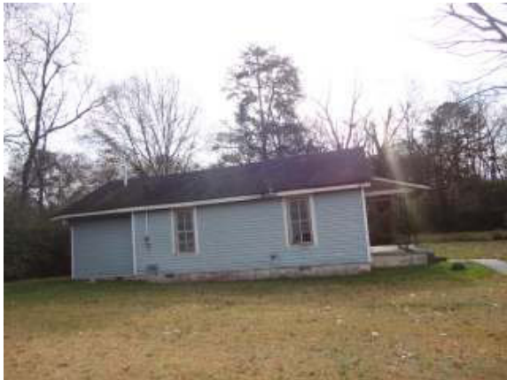
Single-family detached home south of Rockdale (AMP 2)
