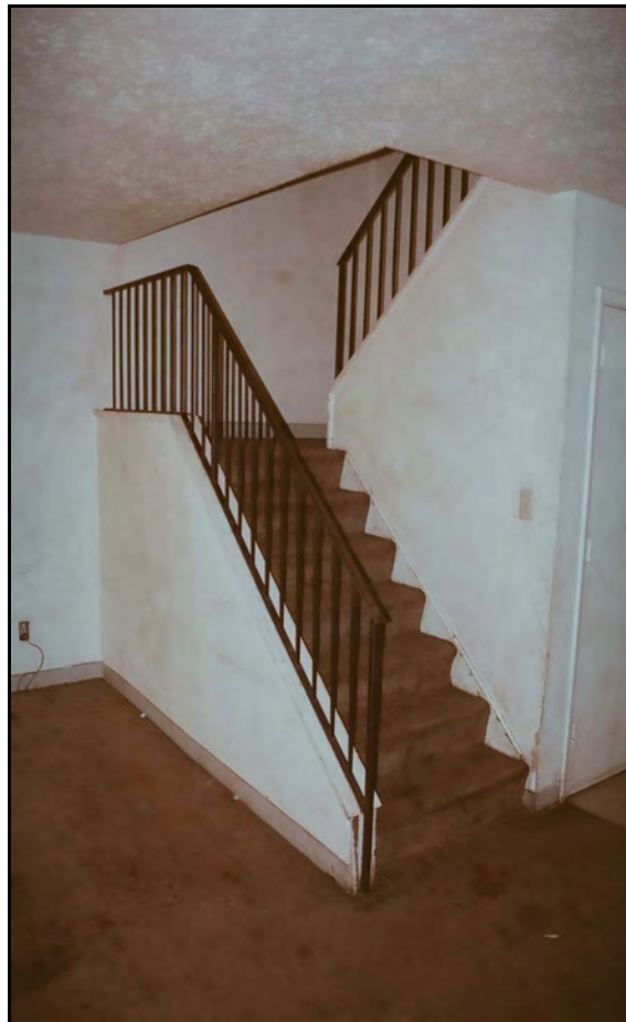
(14) AC Condensers Units & (15) Townhouse Stairway
