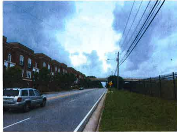
Street view Peachtree Road facing west
