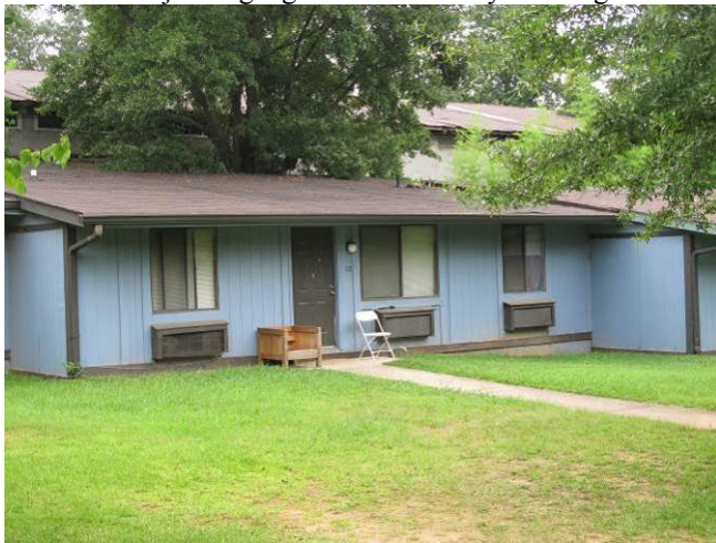
Subject one-story residential building
