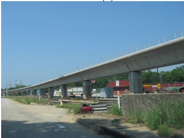
Freight rail line/MARTA rail line along Murphy Ave SW
