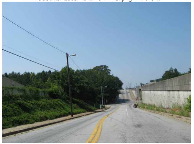
View south on Murphy Ave SW
