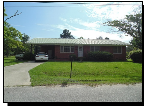
(6) Single-family home off N Gordon Ave, site behind.
