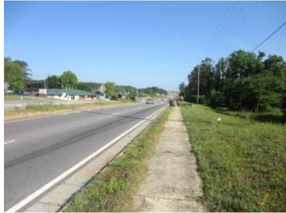
Buford Highway (State Highway 20) looking northwest (site on the right)
