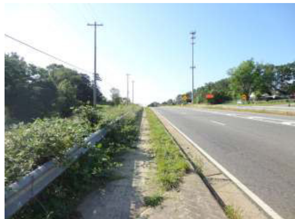
Buford Highway (State Highway 20) looking southeast (site on the left)
