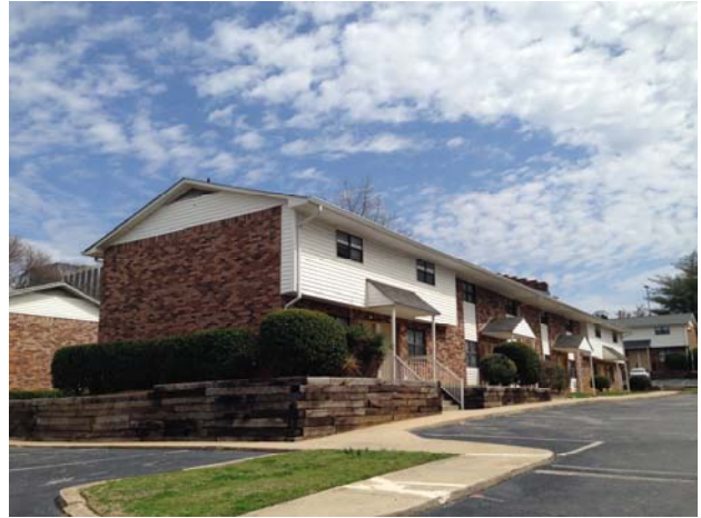
Subject site (to be razed)
