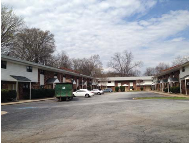
Subject site (to be razed)
