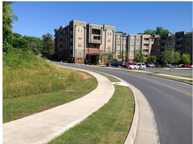
View northwest along Etowah Terrace
