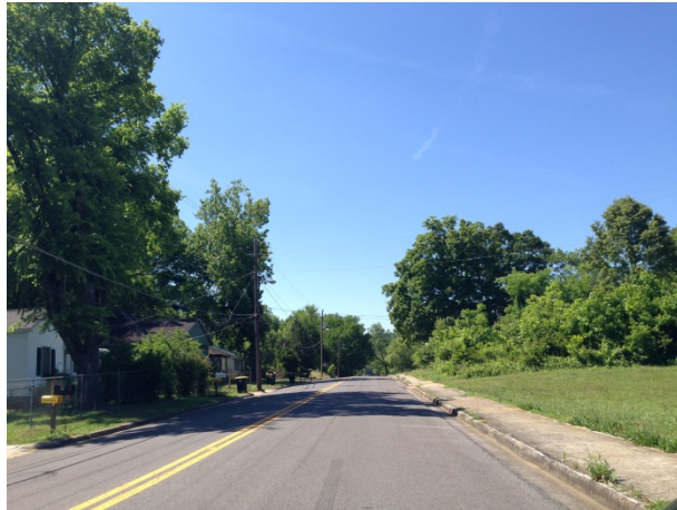
View along Hardy Street facing south
