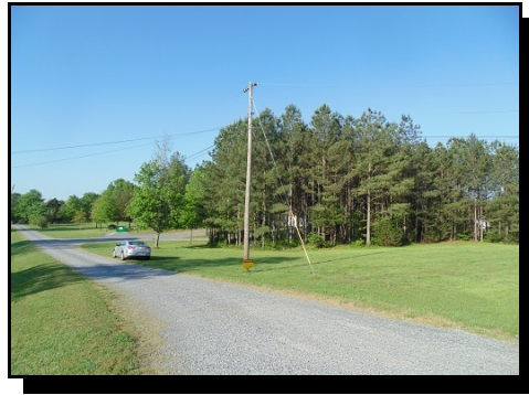
(6) Diagonal view of site, northeast to southwest.
