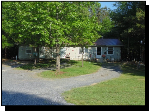
(9) Tri-plex on site.
