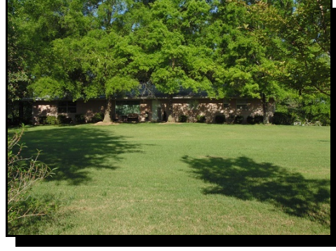
(8) Single-family dwelling on site.
