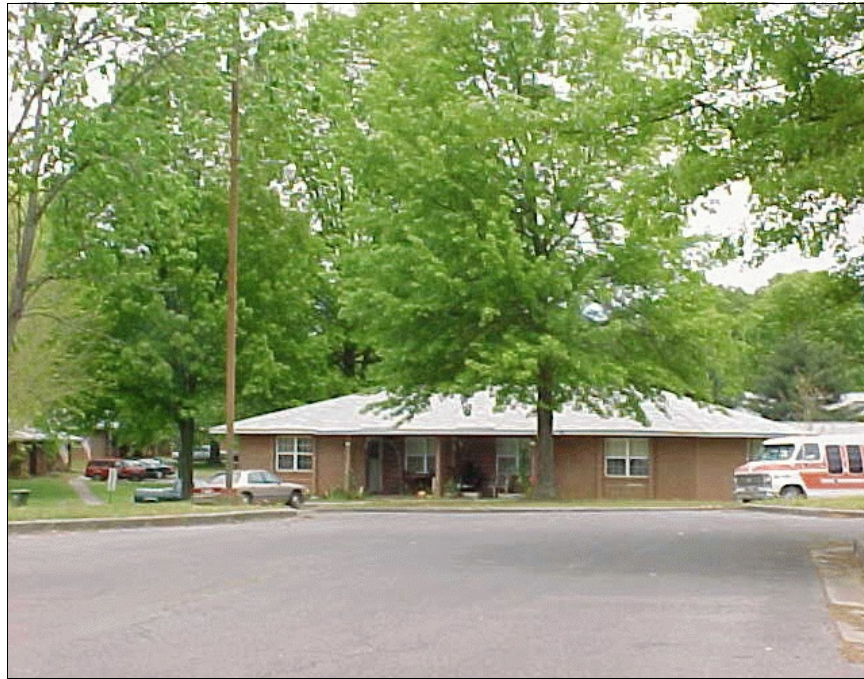
Typical PHA building in Chatsworth.
