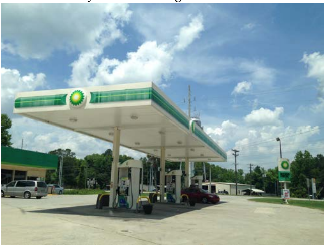
Gas Station along Butler Avenue
