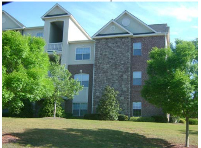
Stonegate at Eagles Landing Apartments north
