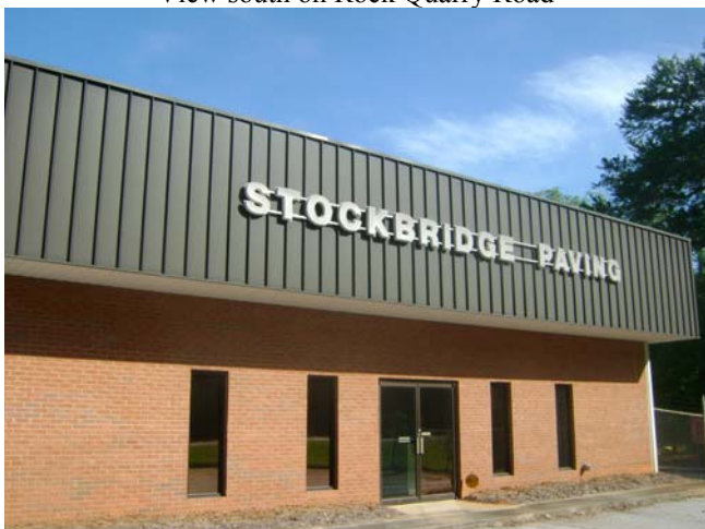
Small commercial development adjacent to site
