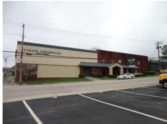
Self-storage facility to the south
