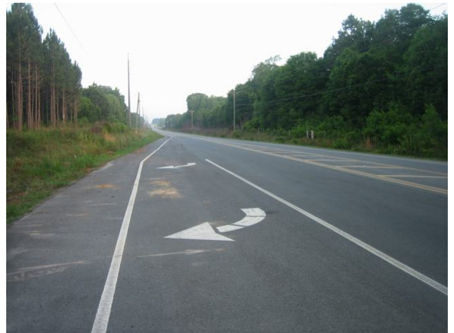
View west on E B Hamilton Drive
