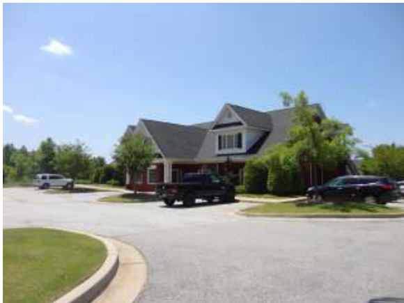
Jefferson City Schools administrative office to the northwest
