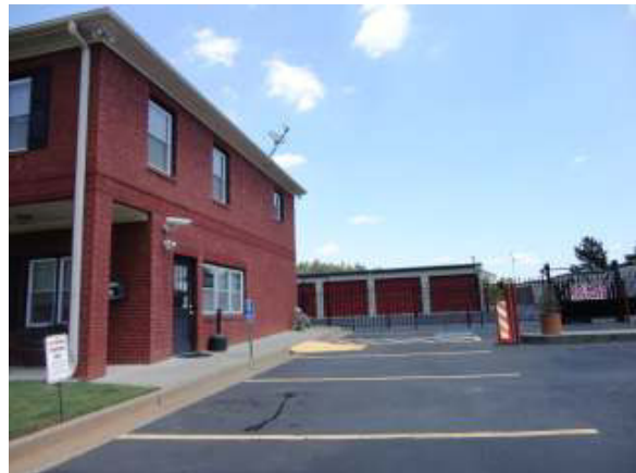
Sunshine Self Storage to the west
