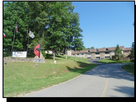
(8) Site behind Methodist Church, south to north.
