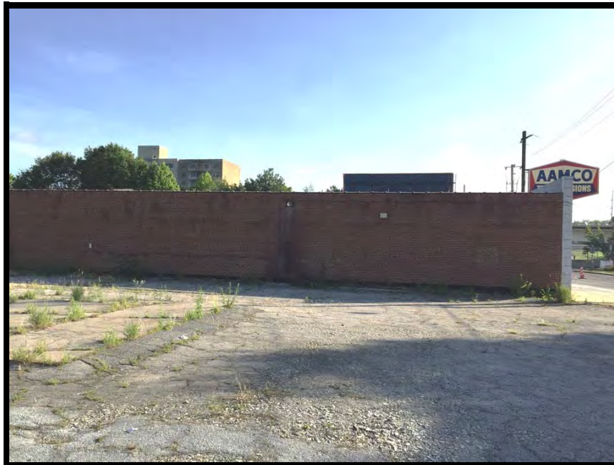
North view from site
