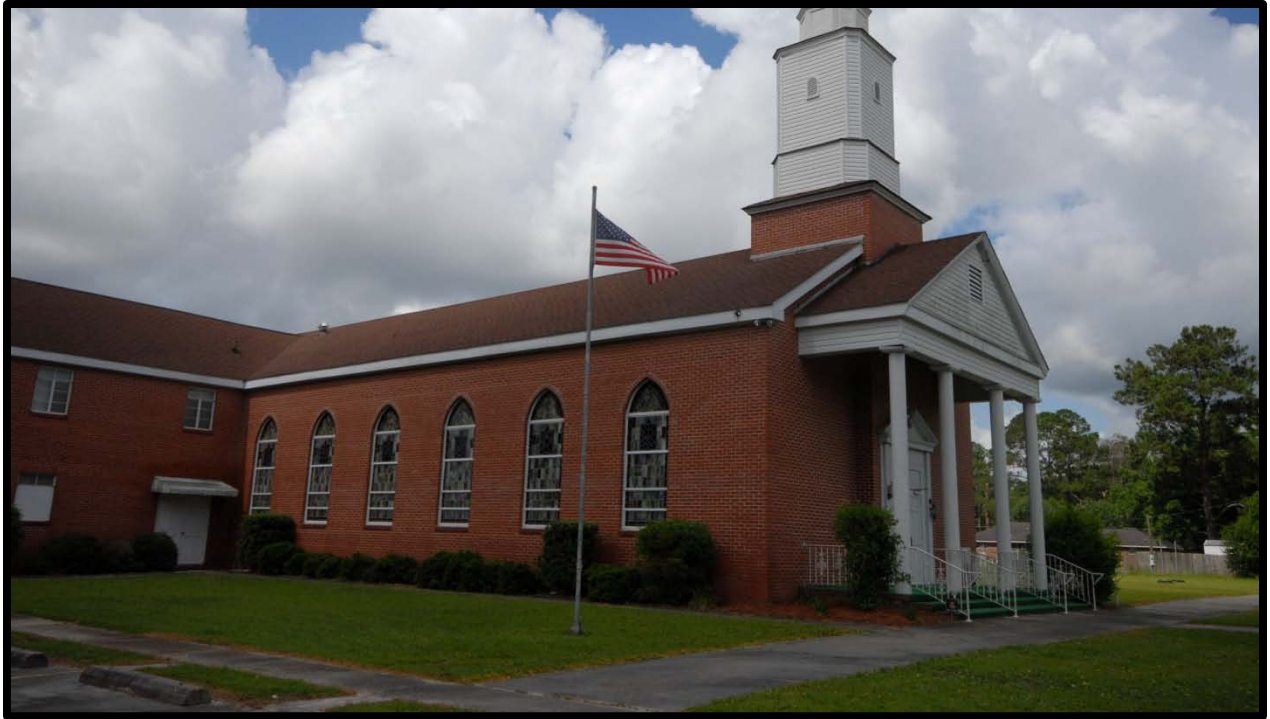
Photo 3 – The church across the street from the site
