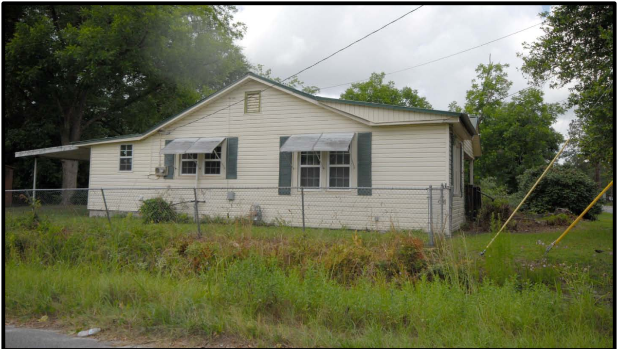
Photo 6 – Home adjacent to the site
