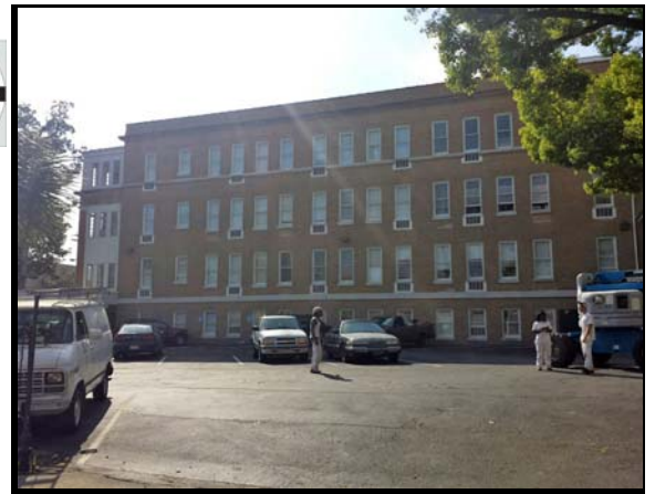
View of site from the east
