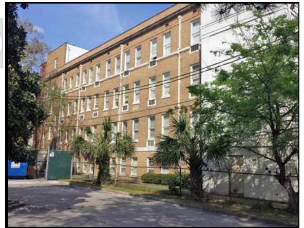
View of site from the west
