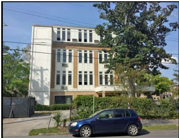
View of site from the south
