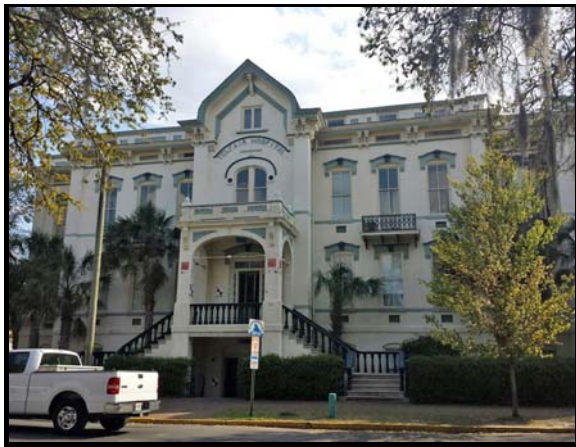
View of site from the north
