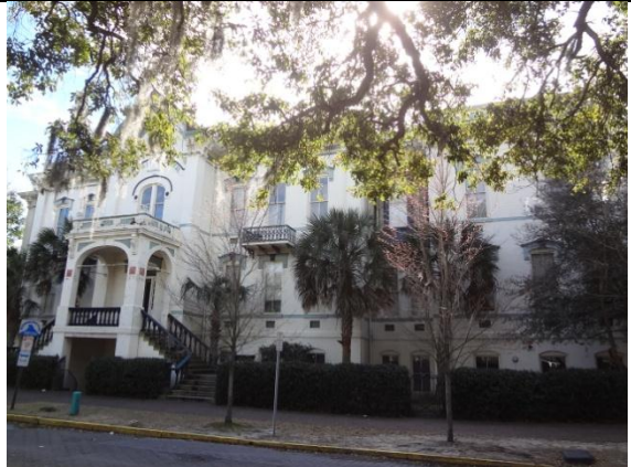
Subject view from Park Avenue
