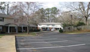
The buildings have a poured concrete foundation. The buildings have a combination brick and siding exterior, and a pitched roof covered with shingles.
