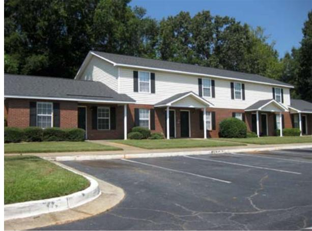
The buildings have a poured concrete foundation. The buildings have a combination brick and siding exterior, and a pitched roof covered with shingles.
