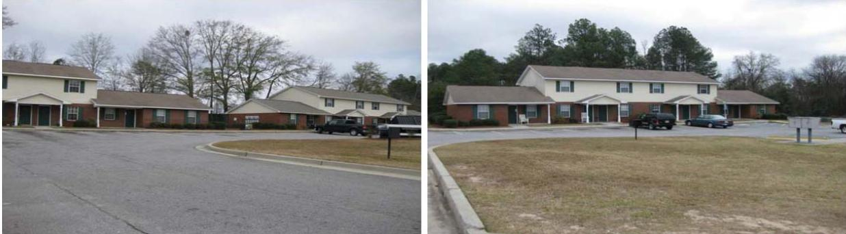
The buildings have a poured concrete foundation. The buildings have a combination brick and siding exterior, and a pitched roof covered with shingles.
