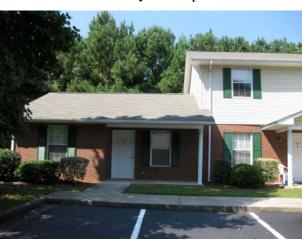
The buildings have a poured concrete foundation. The buildings have a combination brick and siding exterior, and a pitched roof covered with shingles.
