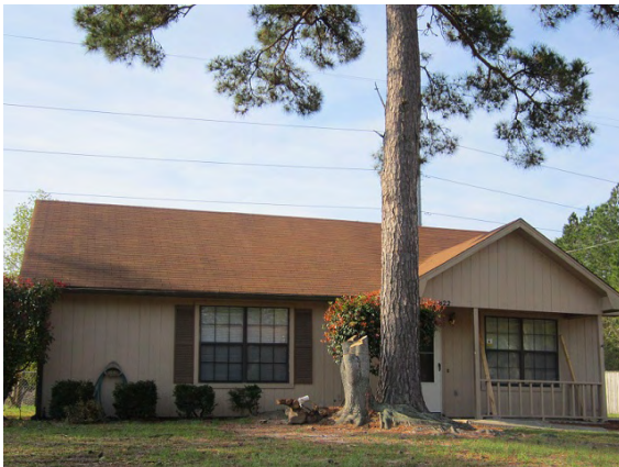
View of a single-family home south of the site
