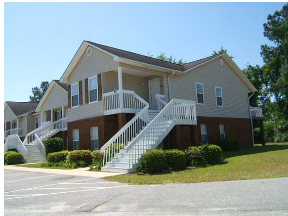
View of Magnolia Plantation Condominiums just east of the site
