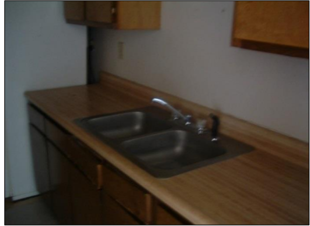
FOUR-BEDROOM UNIT KITCHEN
