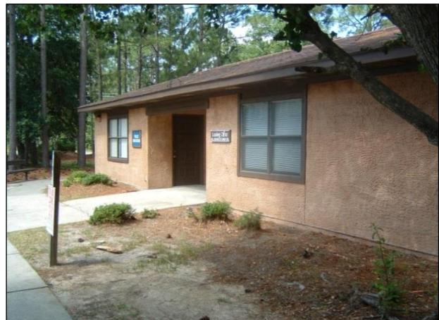
MAIN OFFICE/TYPICAL EXTERIOR
