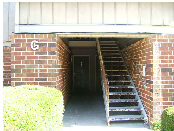
View of an exterior stairwell providing access to the units
