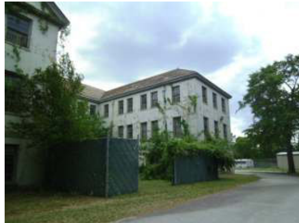
View of building 76 facing southwest
