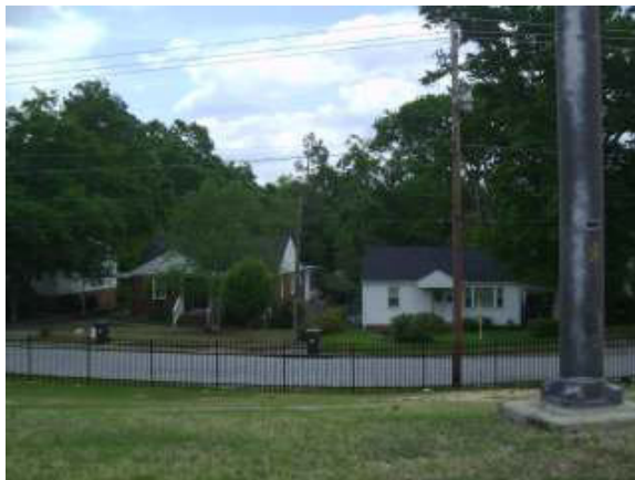
View of a single-family detached homes on Maryland Avenue
