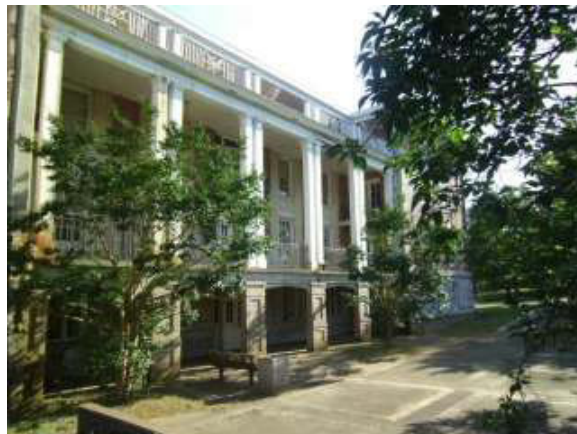
View of northern side of building 18
