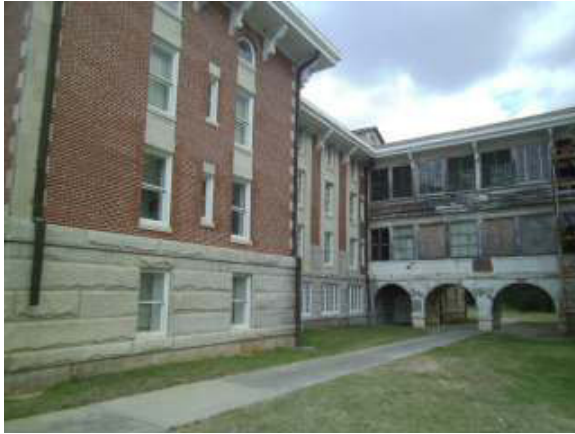
View of building 18 facing northeast
