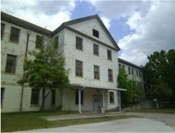
View of building 76 facing northeast
