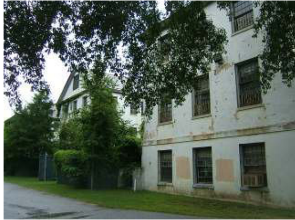
View of building 76 facing north
