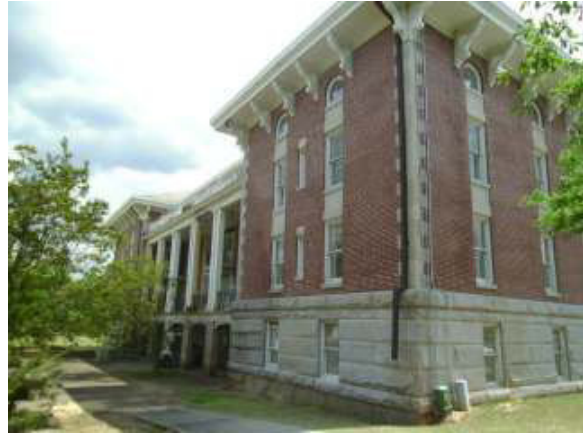
View of building 18 facing southeast
