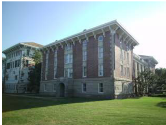
View of building 18 facing southwest
