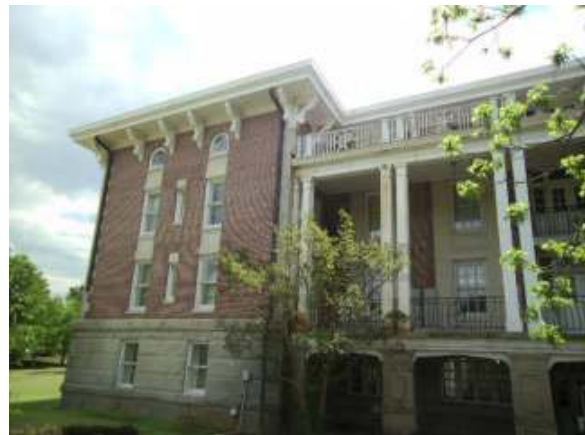
View of building 18 facing south
