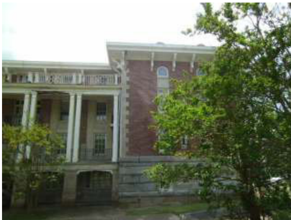
View of building 18 facing south
