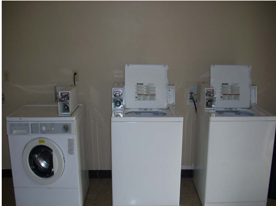
View of Laundry Facility
