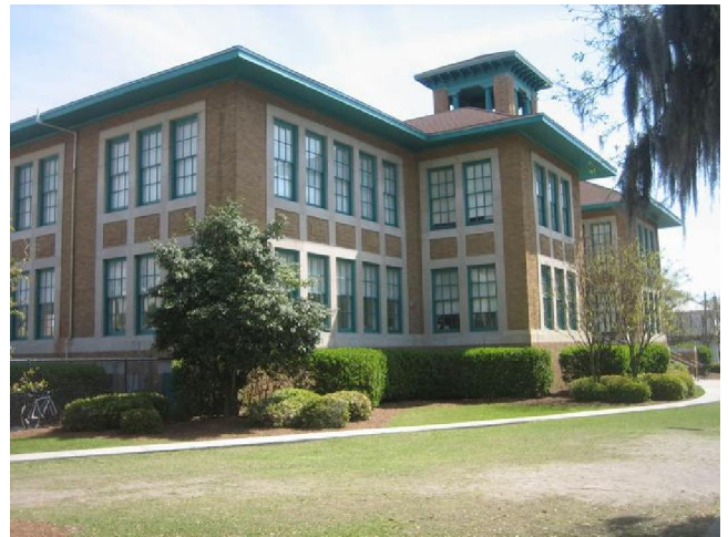
View of SCAD school building east of Subject across Lincoln Street
