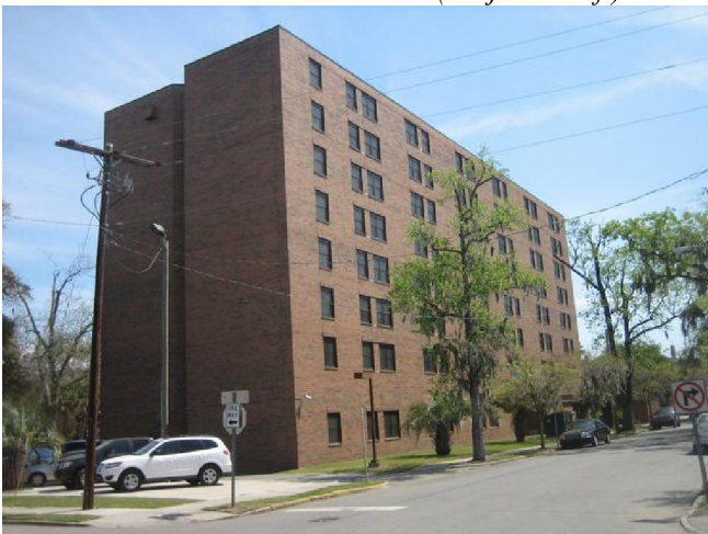
Williams Court northeast of the Subject on East 36 th Street
