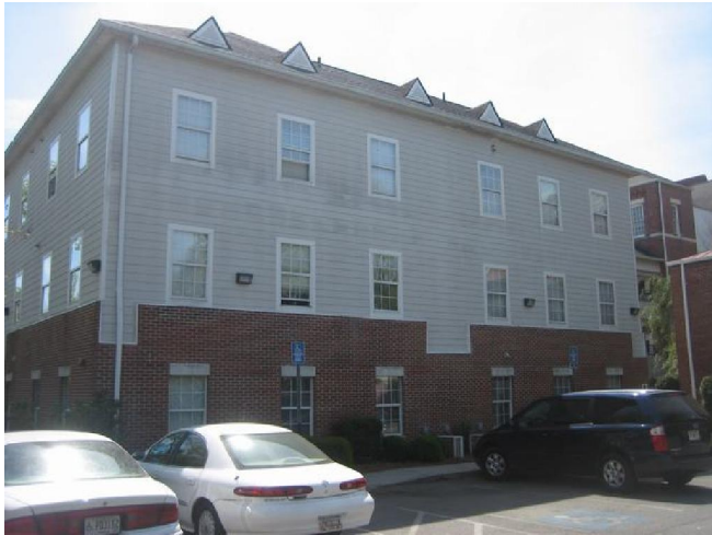
Subject exterior (building will be razed as part of renovation)
