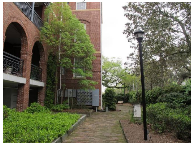
Subject – Brick walking path around the building
