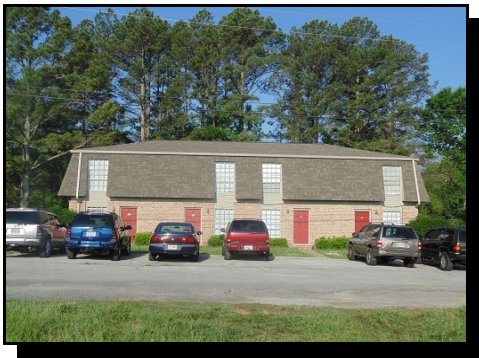
(11) Paxton Place from site, east to west.
