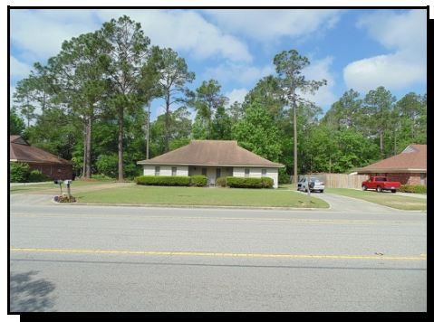
(12) Lester Road Duplexes, north of site.
