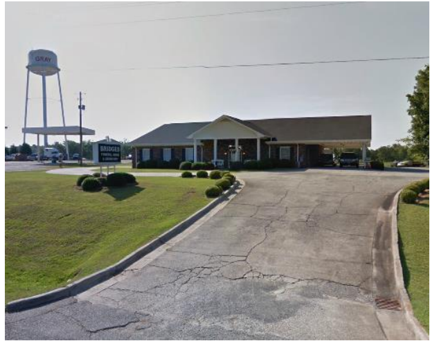
Funeral Home North of Subject Site on Gray Highway
