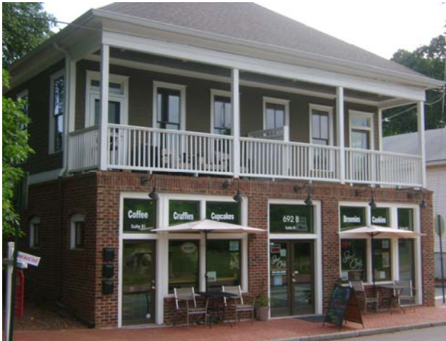
Mixed use development west
