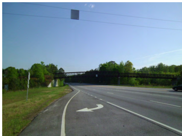
Hwy 278 facing north near site, Silver Comet bridge in background
